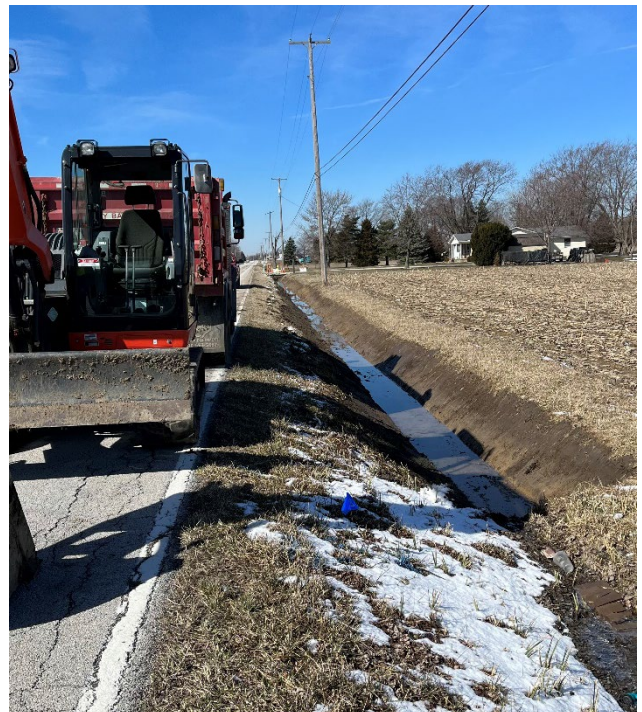
Digging out ditch on CR 247
