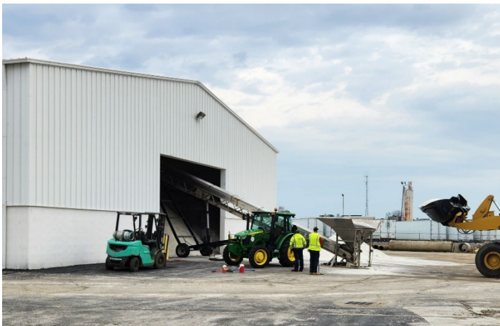
Stacking salt with ODOT's conveyor
