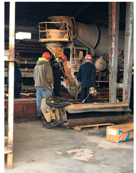
Concrete pouring for the RY 260 – 4.42 bridge beams
