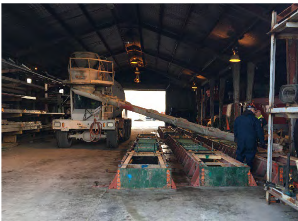
Concrete pouring for the RY 260 – 4.42 bridge beams
